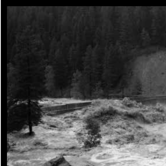
From the old Belton Bridge over the Middle Fork of the of the Flathead River, first day of the flood. (Photo by W.S. Keller.)
