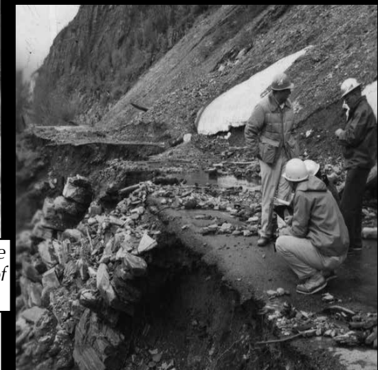
Claude Tesmer, Clarence Bengtson, Charles Riebe and Irv Lloyd inspecting Damage damage on Going-to-the-Sun Road after the 1964 flood (Photo by W.S. Keller.)
