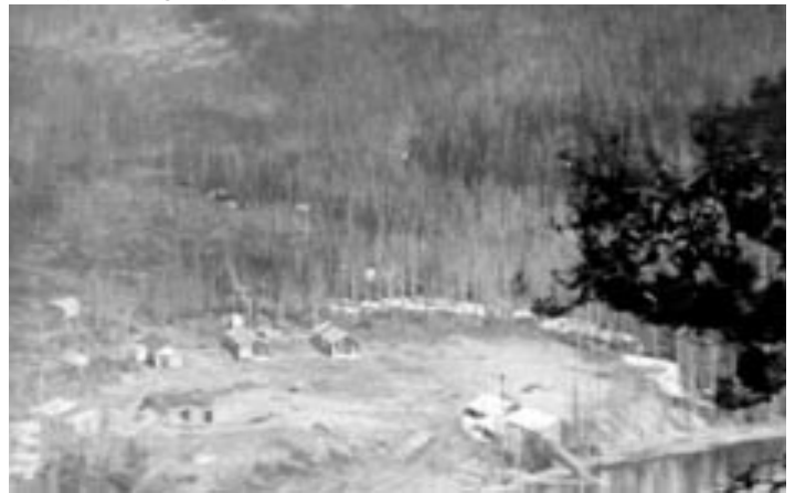
The Many Glacier construction camp, 1914. (Ray Sleeper photo)
