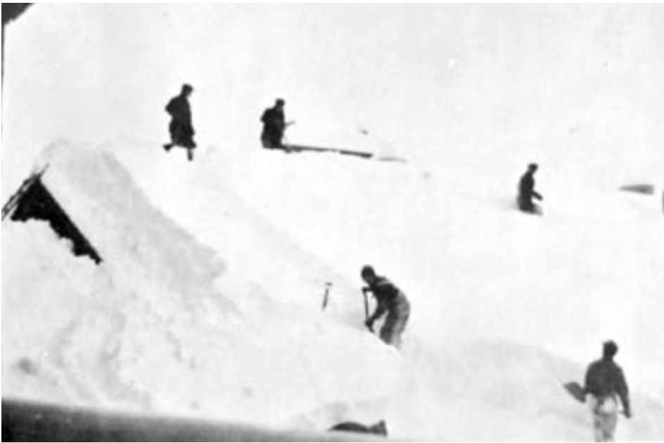
Clearing snow from the roof of Many Glacier Hotel. (Ray Sleeper photo)
