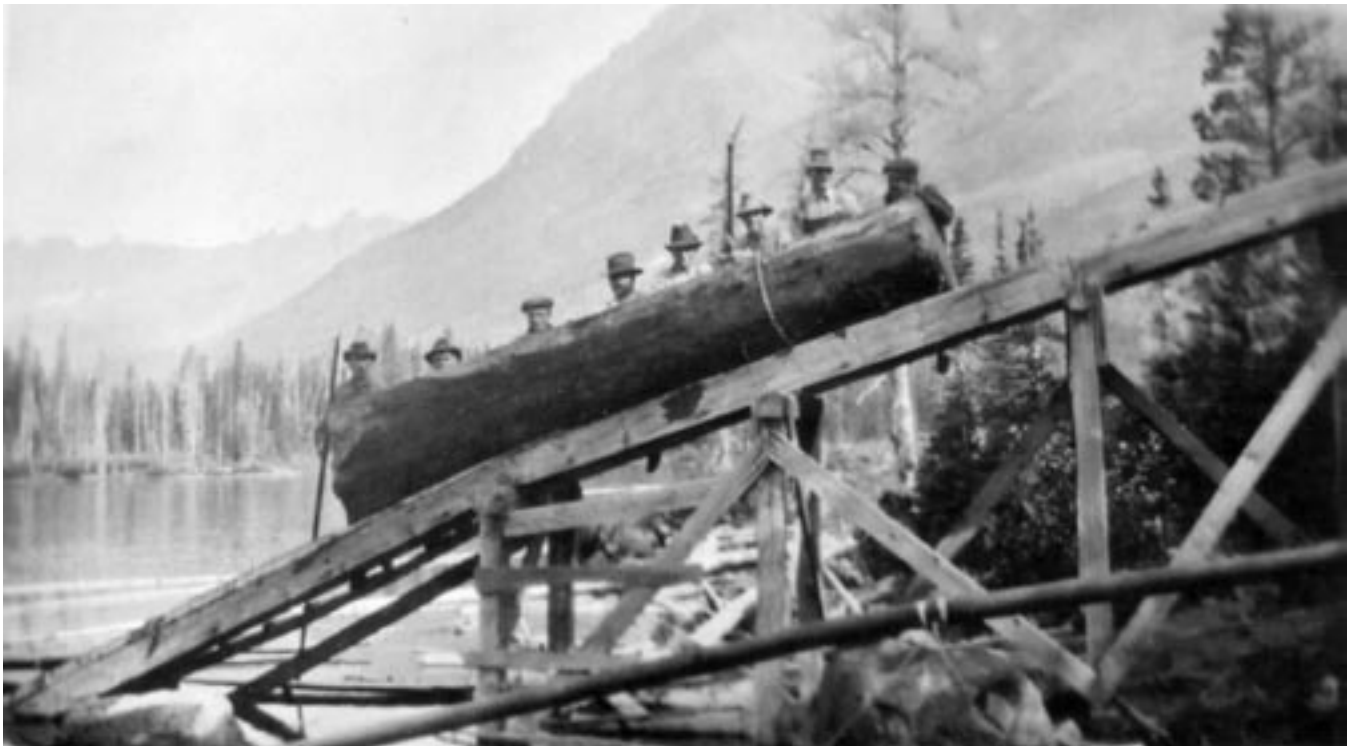
Ramp used to transport logs harvested in the Grinnell Valley to the sawmill at the Many Glacier Hotel construction site, 1914. (Ray Sleeper photo)
