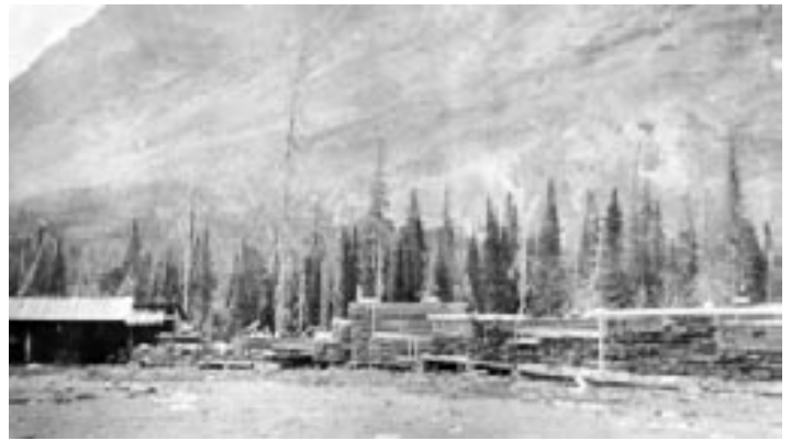
Lumber piled for use in the construction of Many Glacier Hotel, 1914. (Ray Sleeper photo)
