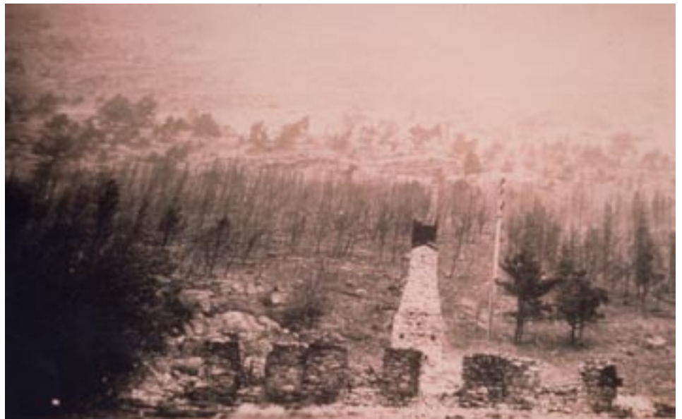
Above: Ruins of one of the Many Glacier chalets, shortly after being burned by the Swiftcurrent Valley fire (Park Service photo).
